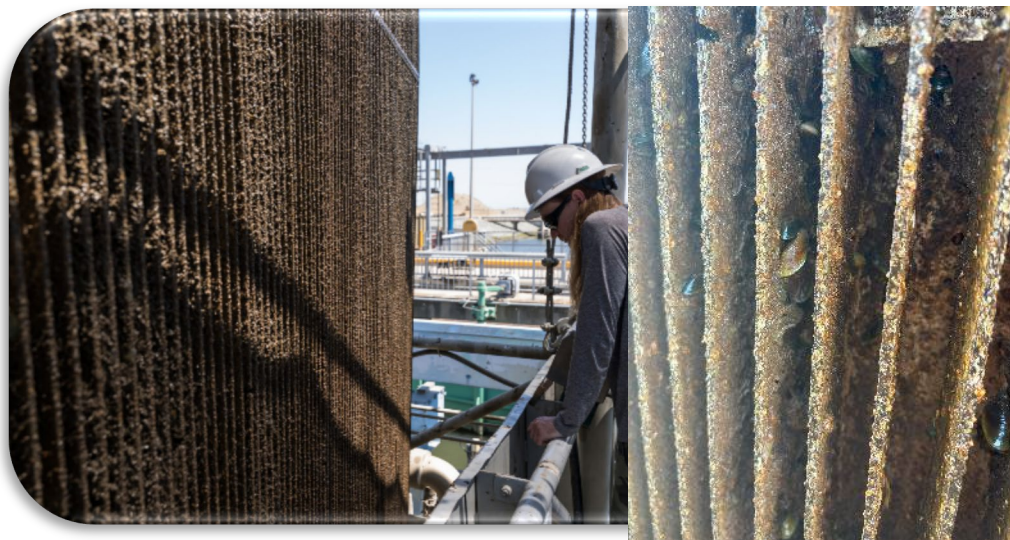
Skinner Delta Fish Protective Facility , Wier
