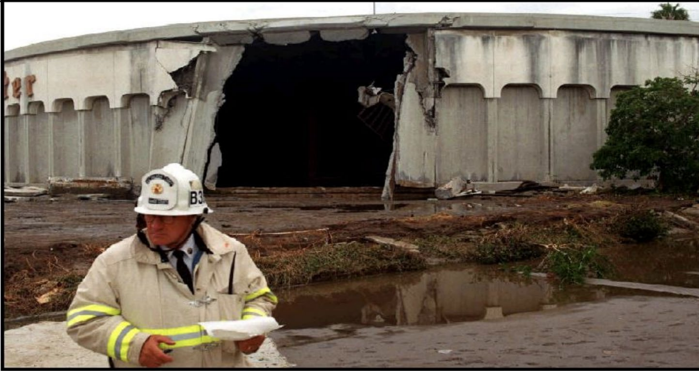
This 31-year-old storage tank ruptured in Westminster, California, sending a 6-foot wave of water through the city that damaged or destroyed about 50 buildings and over a dozen vehicles. Storage tanks should be replaced or periodically rehabilitated to preserve their structural integrity.
