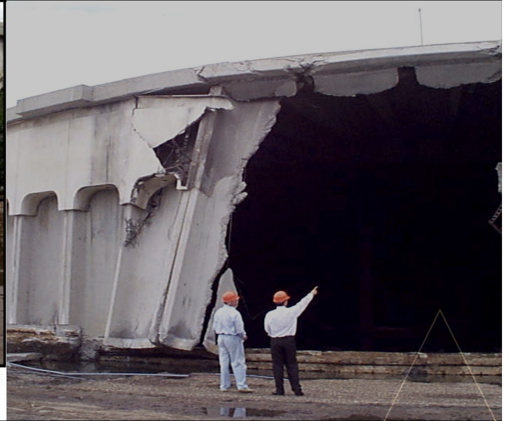
This 31-year-old storage tank ruptured in Westminster, California, sending a 6-foot wave of water through the city that damaged or destroyed about 50 buildings and over a dozen vehicles. Storage tanks should be replaced or periodically rehabilitated to preserve their structural integrity.
