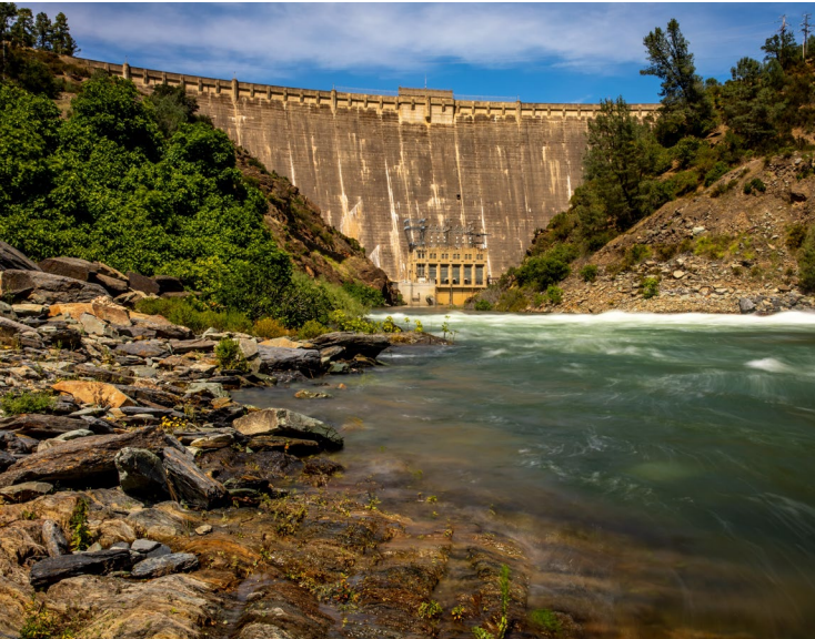
Pardee Dam and Powerhouse
