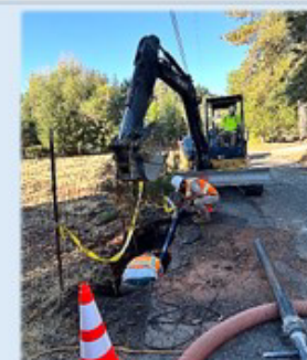
Meadowbrook Line Break Repair
