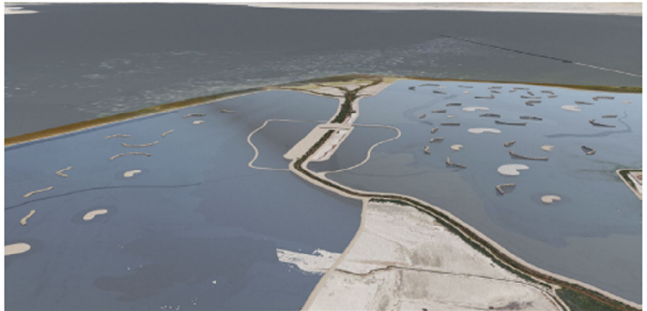
Figure 4. Computer generated imagery of the SCH Project, looking toward the New River Delta. Shown are the habitat ponds to be created on the east and west of the New River, including islands of different shapes to provide avian nesting and loafing sites.
